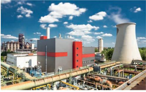
Off gases at ArcelorMittal Eisenhüttenstadt flow (left to right) through the green tubes, directly to the boilers of the external power plant.
