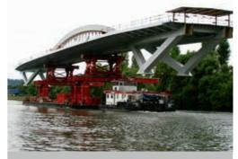
Transport of the bridge's central span by lighter along the Moselle.
