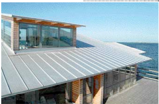
Standing seam roof on the Swedish coast – Lindab Buildings
