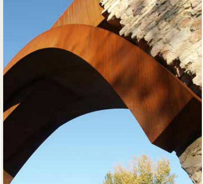
Restoration of the Trençat Bridge, Sant Celoni, Spain Design and engineering: Xavier Font - Alfa Polaris S.L. Copyright picture: Xavier Font
