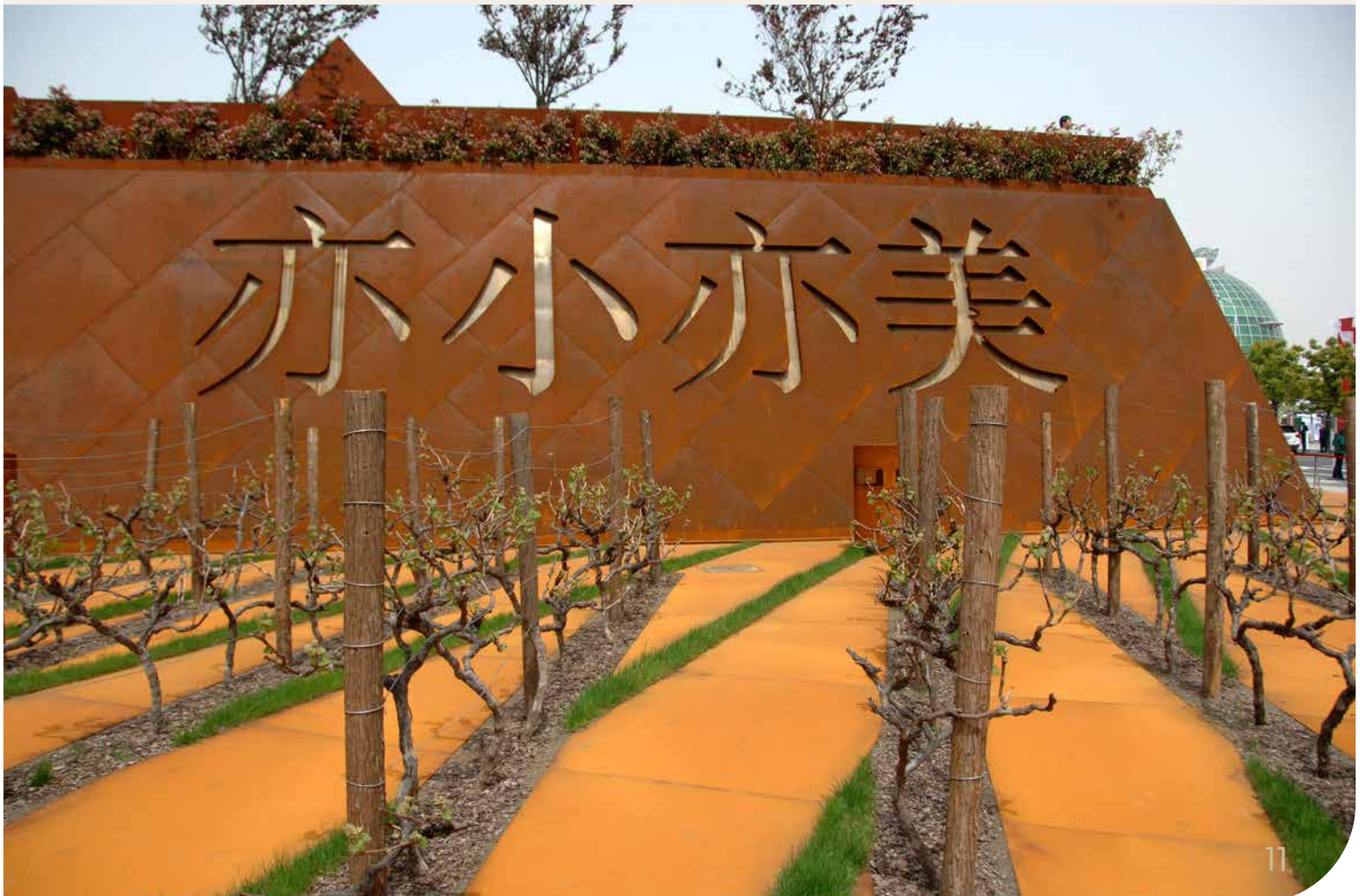
Luxembourg's national pavilion at the 2010 Shanghai Expo, China / Architect: Hermann & Valentiny et Associés Copyright picture: ArcelorMittal / Pierre Engel
