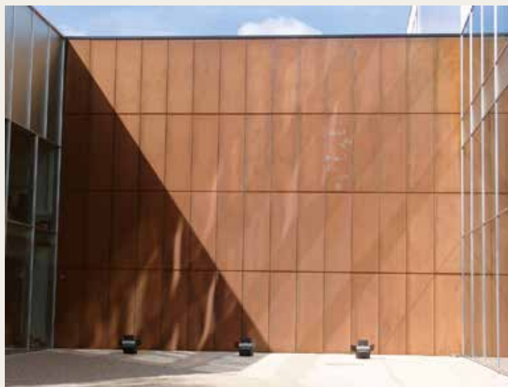
Metal Structures Centre (MSC), Gent, Belgium Copyright pictures: Gert De Vos
